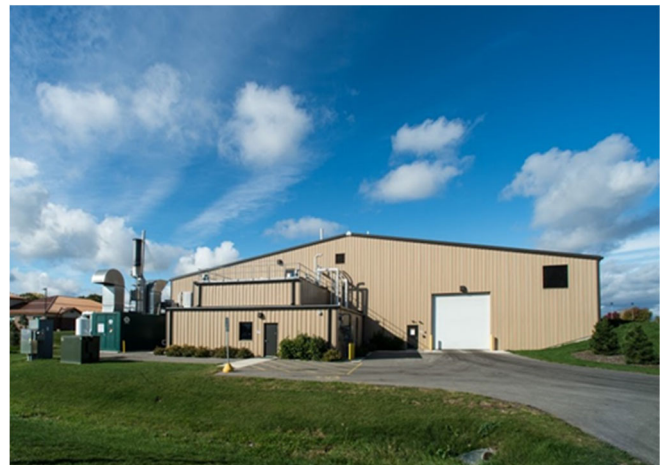
General view of the site: the CHP unit can be seen on the left. The large white door is the entrance to the bay area and the AD chambers
