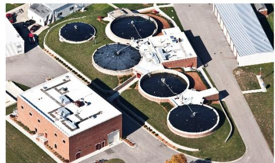
Four 55 Ft Diameter Digesters plus 40 Ft Digested Sludge Storage Tank (source KWRD)
