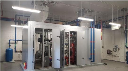
CHP Unit 1 – 375 kW Biogas Fueled Sys
