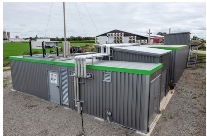
General view of the site: two fermentation vessels, biogas storage pump room, feedstock transfer building, technology research lab, control room, CHP unit
