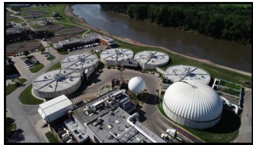
Digester Complex Des Moines WRF Source: Des Moines Wastewater Reclamation Authority
