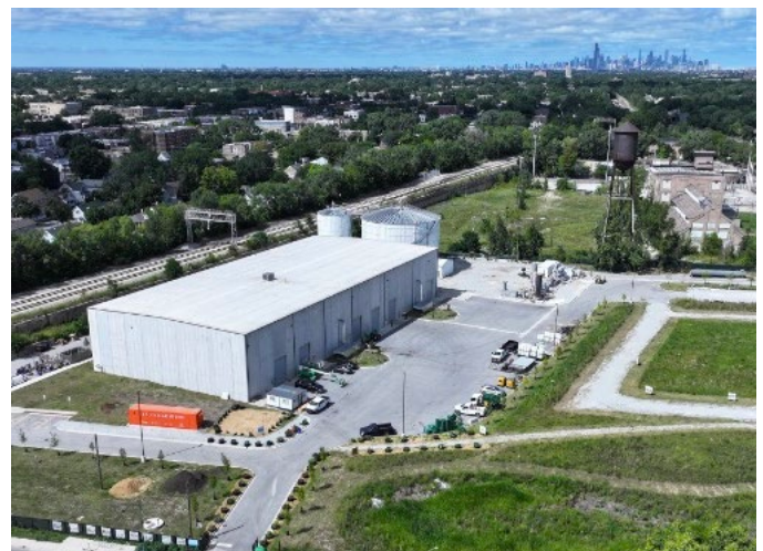
The Green Era Campus in construction
